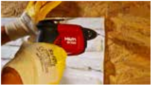
4-b) Assembling by screws
