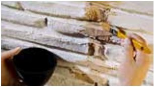
8- Whiping into shape by brush and putty knife
