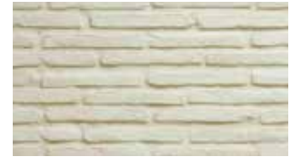
11- Installation finished after drying
