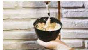
6- Preparing the assembly putty
