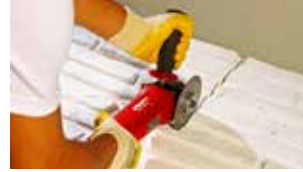
3- Cutting the panel by angle-grander
