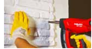
4-a) Assembling by nails
