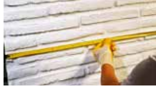
2. Scaling of the panel to be applied
