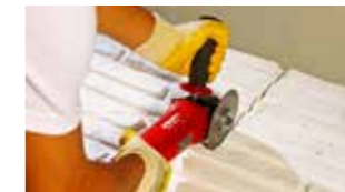
3- Cutting the panel by angle-grander
