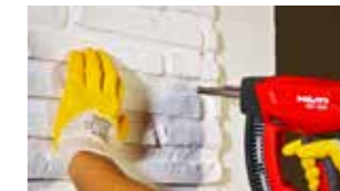
4-a) Assembling by nails
