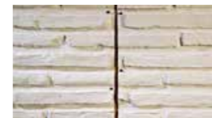
5- Leaving a space by 1cm between two panels
