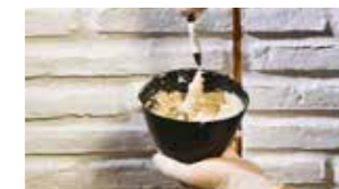
6- Preparing the assembly putty
