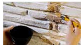
8- Whiping into shape by brush and putty knife
