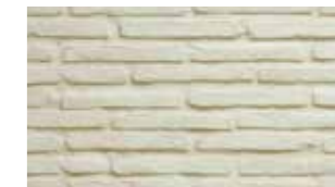
11- Installation finished after drying
