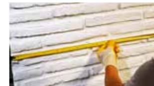
2- Scaling of the panel to be applied
